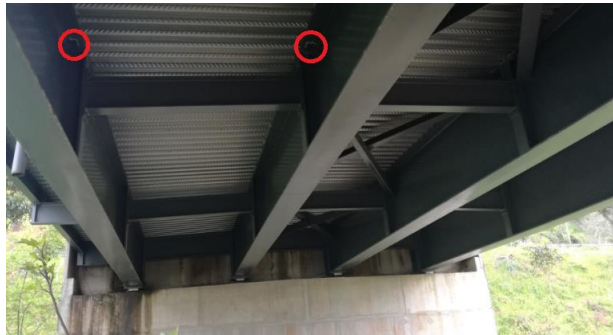
Figure 3: Visible extensometers (strain gauges).
