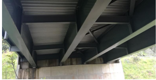
Figure 2: Profiled sheet, longitudinal and cross girders.
